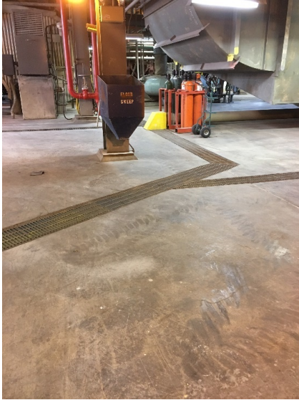
Photo 4-9 Blowdown Drain Pipe Routing to Sump
