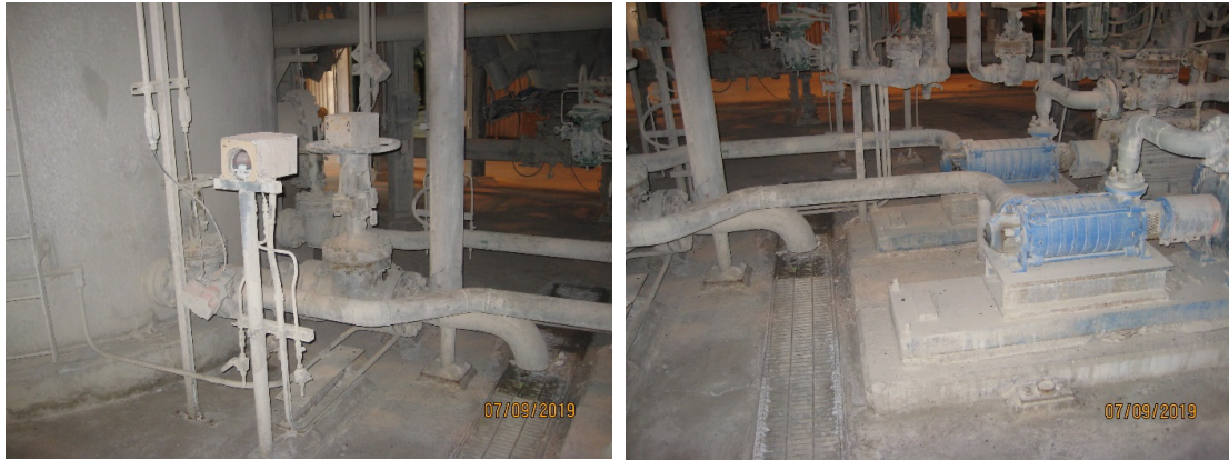
Photo 4-7 Photos Showing Cooling Water Pump Suction Strainers Removed
