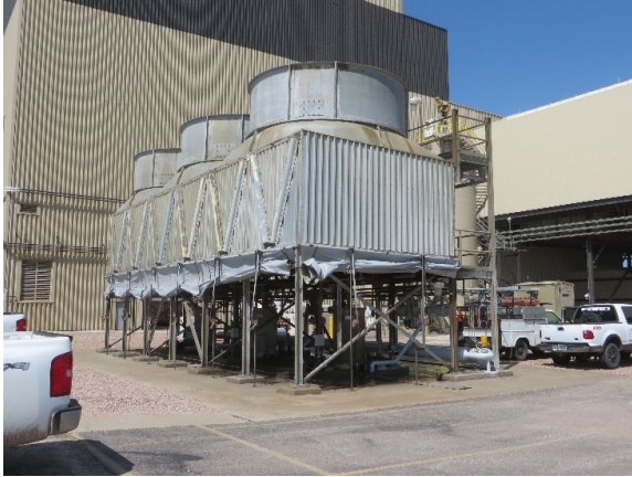
Photo 4-4 Old Auxiliary Cooling Tower
