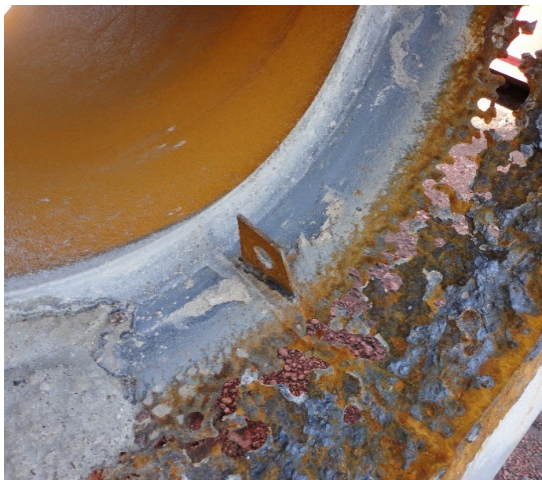
2011 photo of the venturi corrosion
