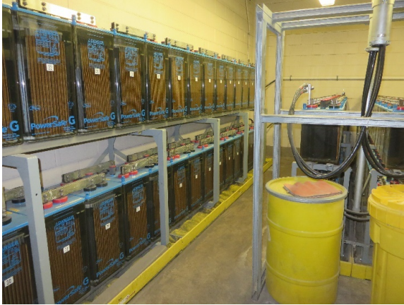
Photo 4-5 UPS Batteries
