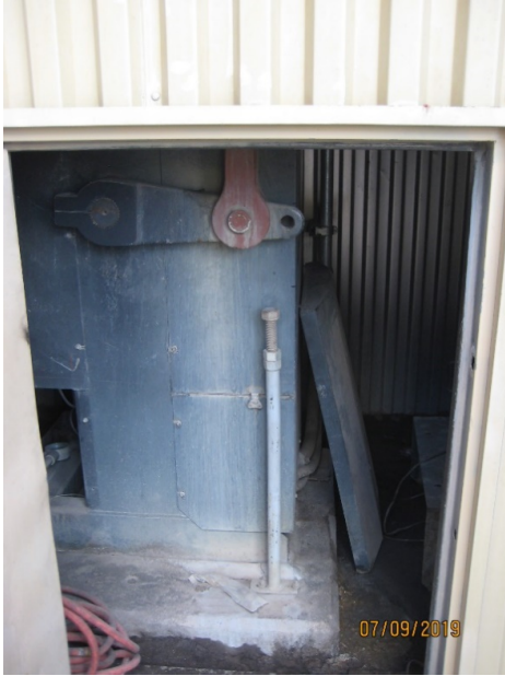
Photo 4-2 Pneumatic Controller for ID Fan VIVs
